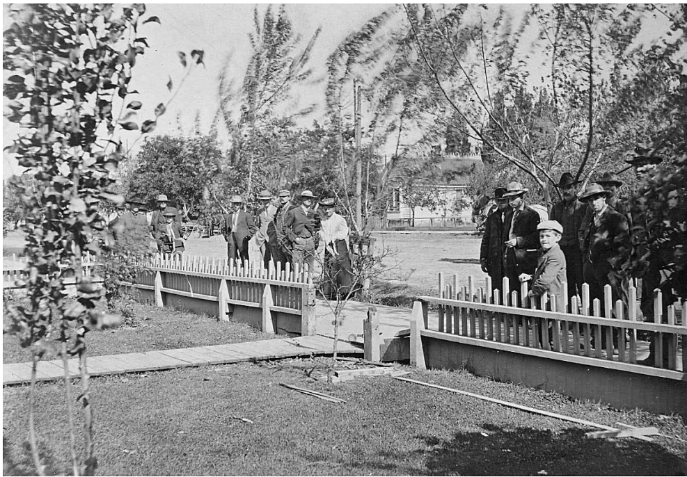
Dynamite bomb was attached to damaged fence post.
